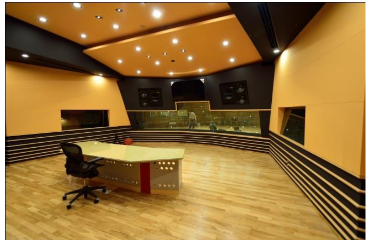
CONTROL ROOM, MASTER CONTROL ROOM
